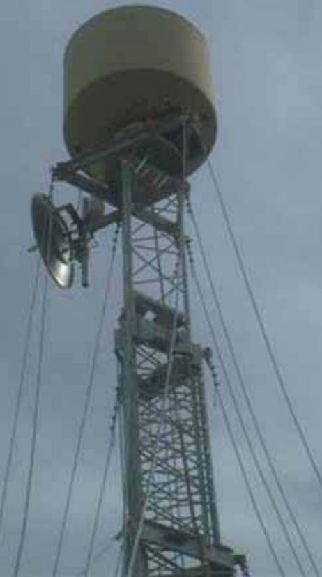
**D**uring the Pre-deployment Site Survey to Operation Enduring Freedom in July 2007, the C Band antenna was elevated to maintain line of sight between the Ground Control Station and the Warrior Alpha aircraft. This was from run up to taxi and then subsequent take off to include climb out to exit down range for the mission.
