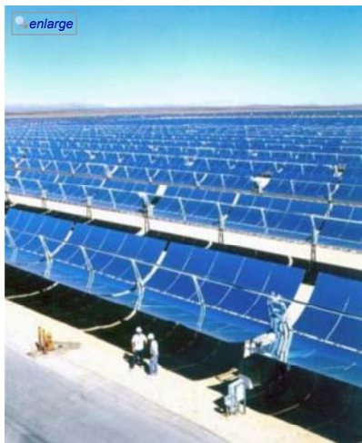
The world's largest solar power facility, located near Kramer Junction, Calif., consists of five Solar Electric Generating Stations and covers more than 1,000 acres. (Credit: Department of Energy/National Renewable Energy Laboratory)
