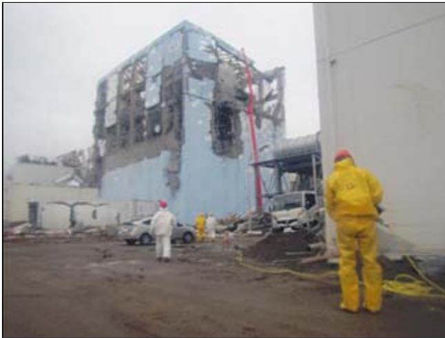
Using a concrete pumping truck, normally used on construction projects, workers were able to spray water into the top of plant No. 4 at Fukushima 1. Photo courtesy of World-nuclear-news.org.
