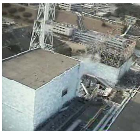
Reactors 2 (left) and 1 (right), April 10, 2011 (TEPCO)
