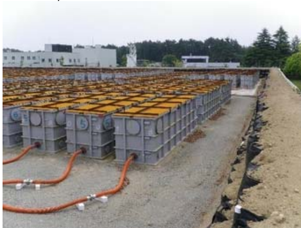
Temporary storage tanks for water with low and intermediate levels of contamination
