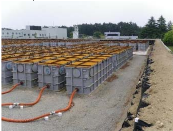
Temporary storage tanks for water with low and intermediate levels of contamination
