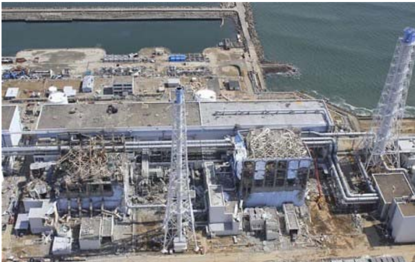
The damaged Unit 3 (left) and Unit 4 Photo: AIR PHOTO SERVICE/AP 9:24AM BST 30 Mar 2011
