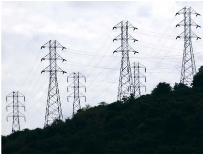
Power line towers. (credit: Getty Images/Justin Sullivan)
