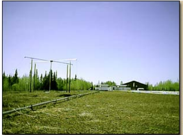
Hipas antenna field, looking toward the transmitter and generator building
